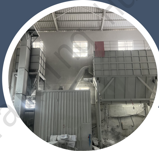
Ring-Roller Grinding Mill Pass Rate: 90% - FULL Pass
